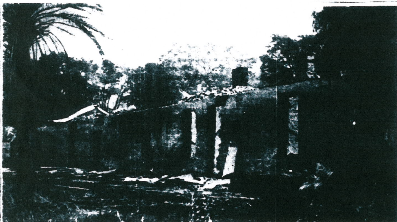
• This is all that was left of the old Manning Estate home in Hamilton-road, Spearwood, after a fire swept through the building early yesterday morning.
